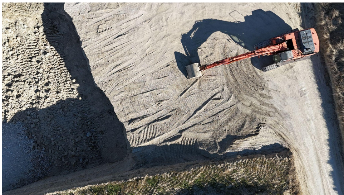
Observation point 3 - Excavated ground pit
