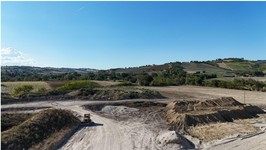
Aerial view of the excavation site( Italy). Source: DJI Mini Pro 4
