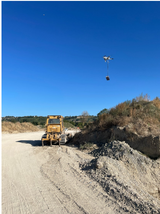
Observation point 1 - Facility entrance
